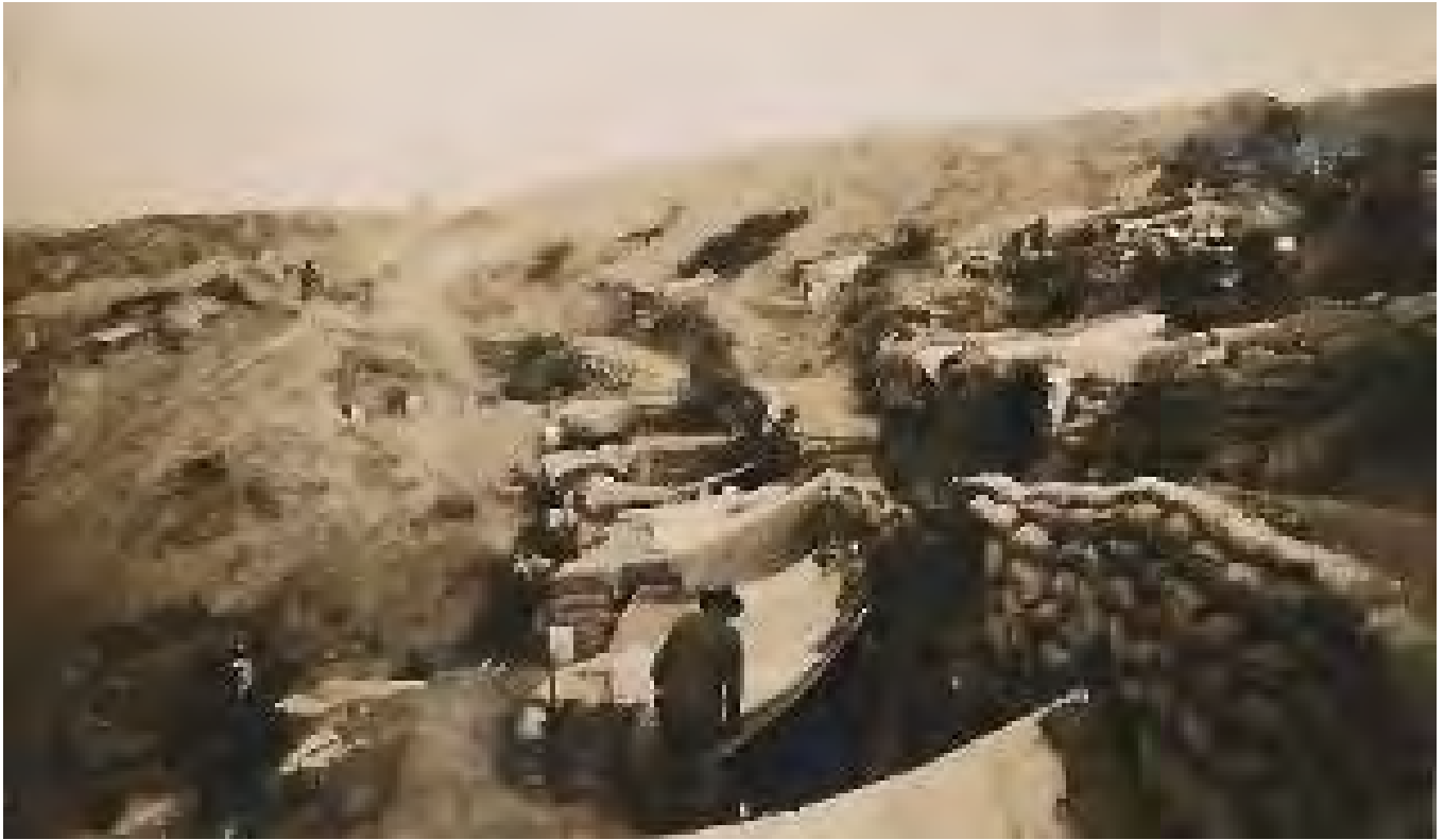
The trenches at Poppy Gully
